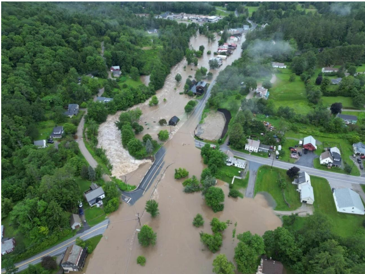
Figure 23 Drone footage of Williams Dam and N Main St 07/11/2023 1
